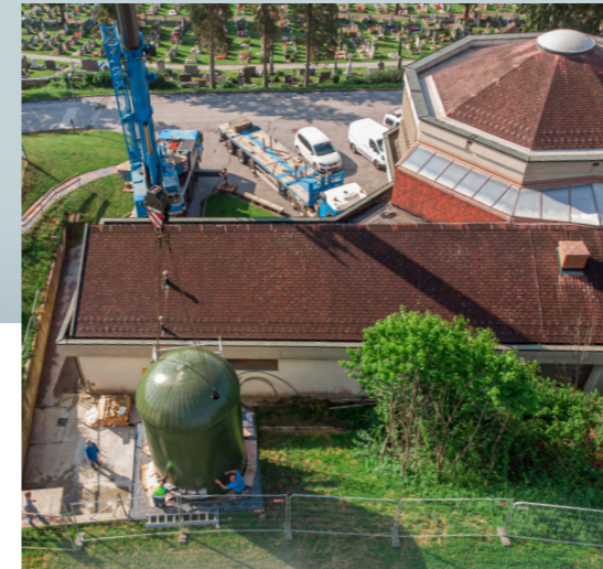
Top left: The Town of Weiz. Top right: The location of the implemented heat storage. On the left: Installation of the new heat storage tank to the heating plant.
