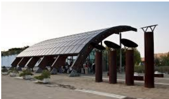
16 kWp PV plant
