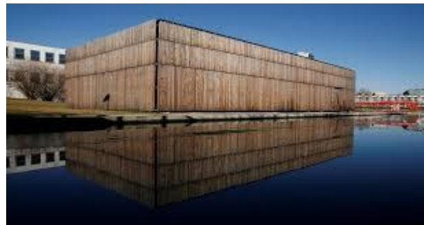
670 kWp hydroelectric plant
